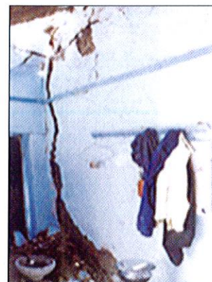
Fig. 5.3 G3 damage (a) Corner Deep & Wide Crack
