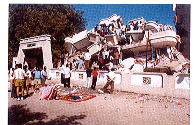
Fig. 5.12 Total Damage G5 of RC Frame Building
