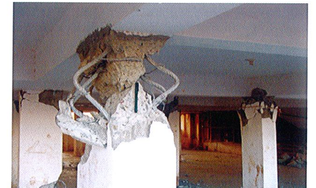
Fig. 5.10 G5 Damage of RC Column
