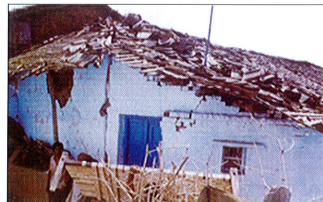
Fig. 5.3 G3 damage (b) Disturbed Tiles on Bricks House
