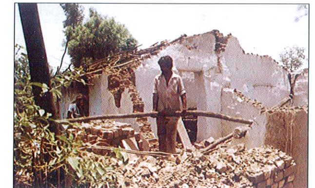
Fig. 5.5 G5 damage Total Collapse
