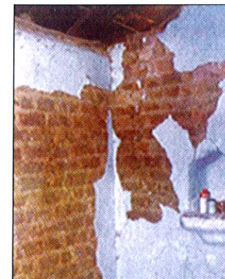
Fig. 5.2 G2 Cracks (c) Large Plaster Spalling
