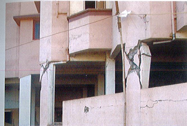
Fig. 5.9 G4 Damage of RC Short Column
