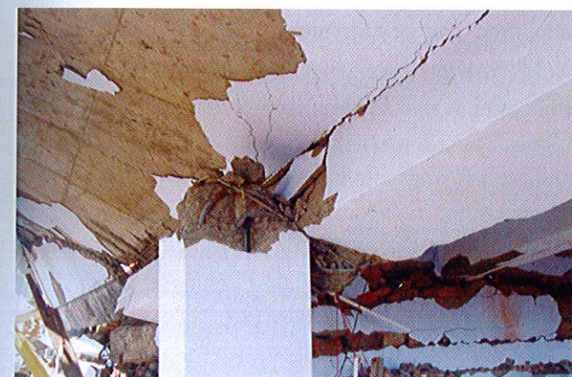
Fig. 5.11 G5 Damage of Beam Column Joint
